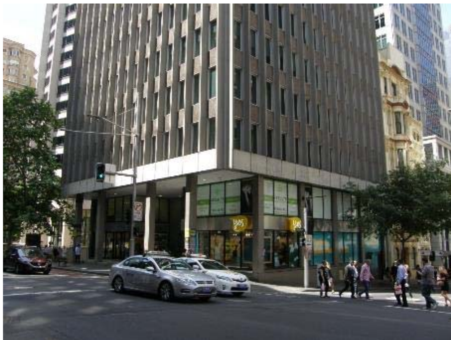
Figure 3 Lower levels of the existing building, note the colonnade located along the George Street frontage of the site.
