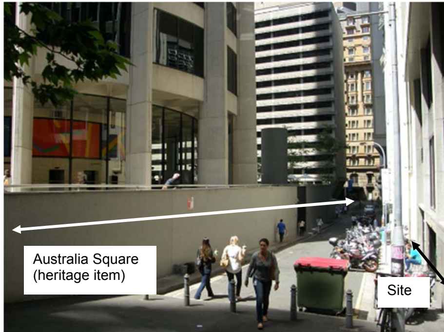
Figure 5 Curtin Place looking east. The heritage listed Australian Square complex is seen on the left hand side of the photograph.
