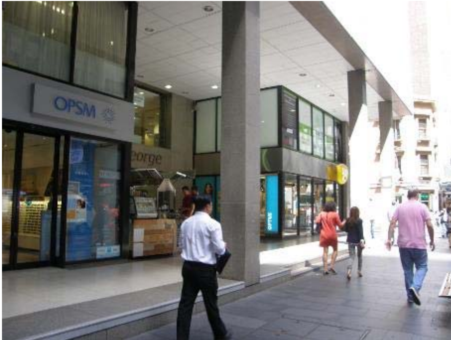
Figure 4 Colonnade along the George Street frontage of the existing building.
