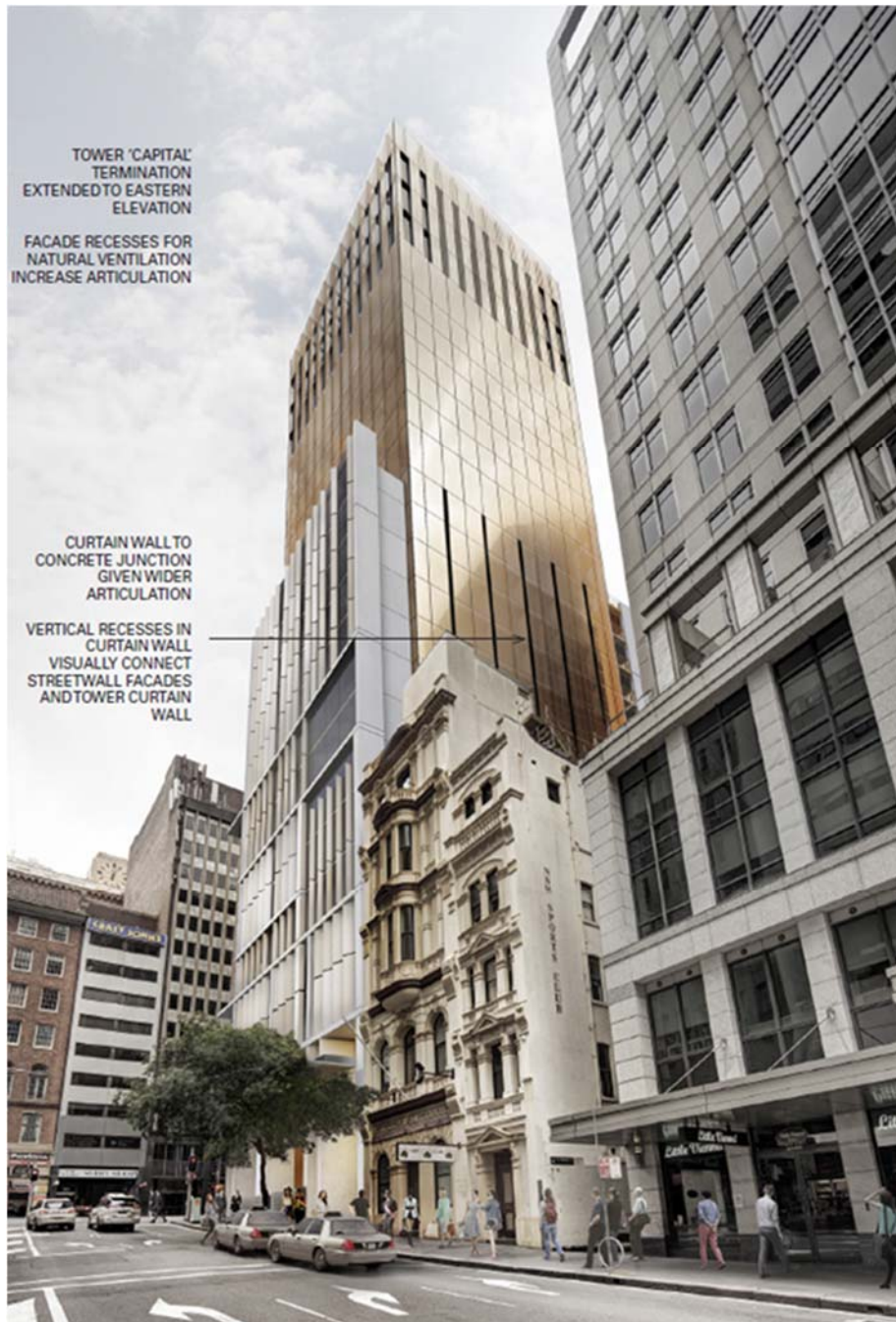
Figure 17 Photomontage showing the relationship between the proposed development and the adjoining heritage listed NSW Sports Club building.
